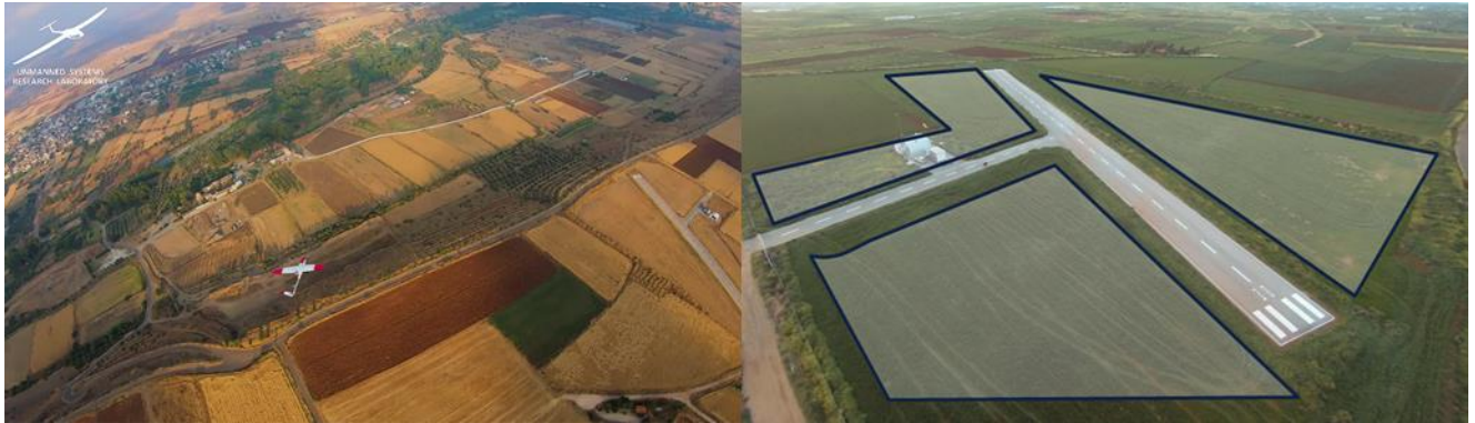
Figure 10 - The CAO-ORO UAV runway and airfield. The three grey areas surrounding the runway in the right photo delimit the land that has been purchased recently.
